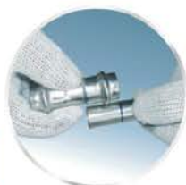
3. Mark the tube for checking the fitting insertion depth size
